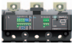
Loose trip unit
